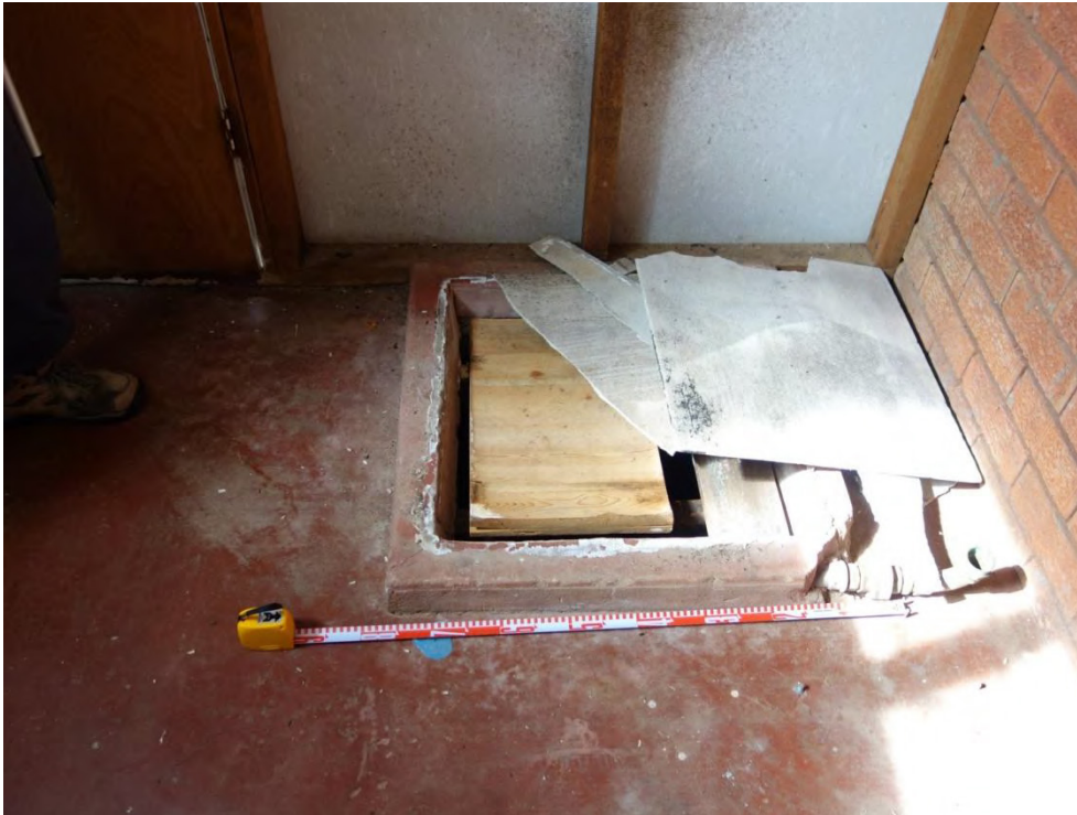
Plate A50 Internal sandstone lined well at 1972 The Northern Road, capped with fibro and timber. (Source: RPS 2015)
