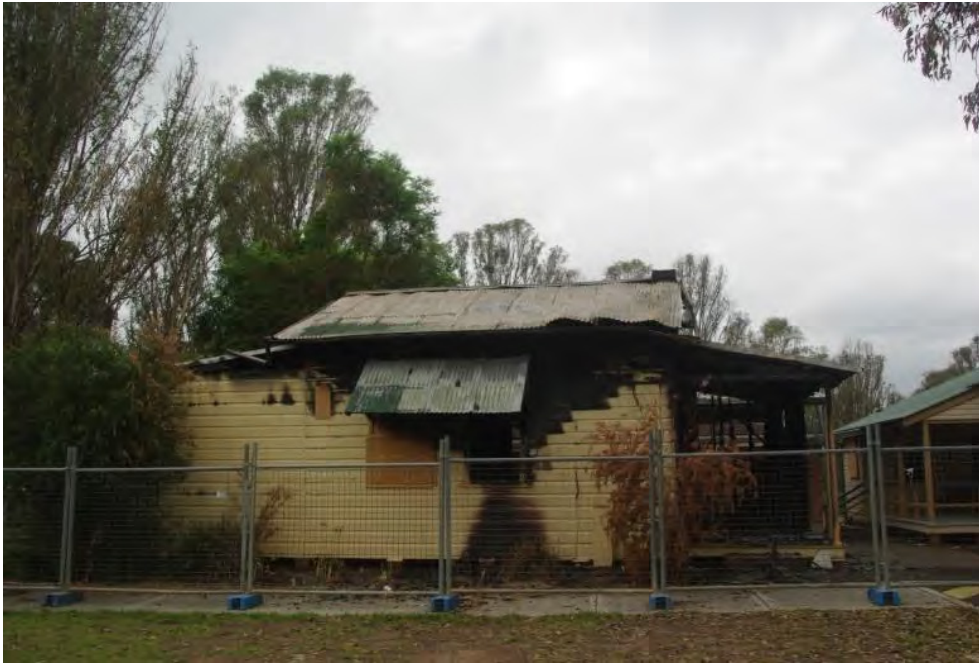
Plate A19 View toward western wall of the staff room, note extensive fire damage. (Source: RPS 2015)
