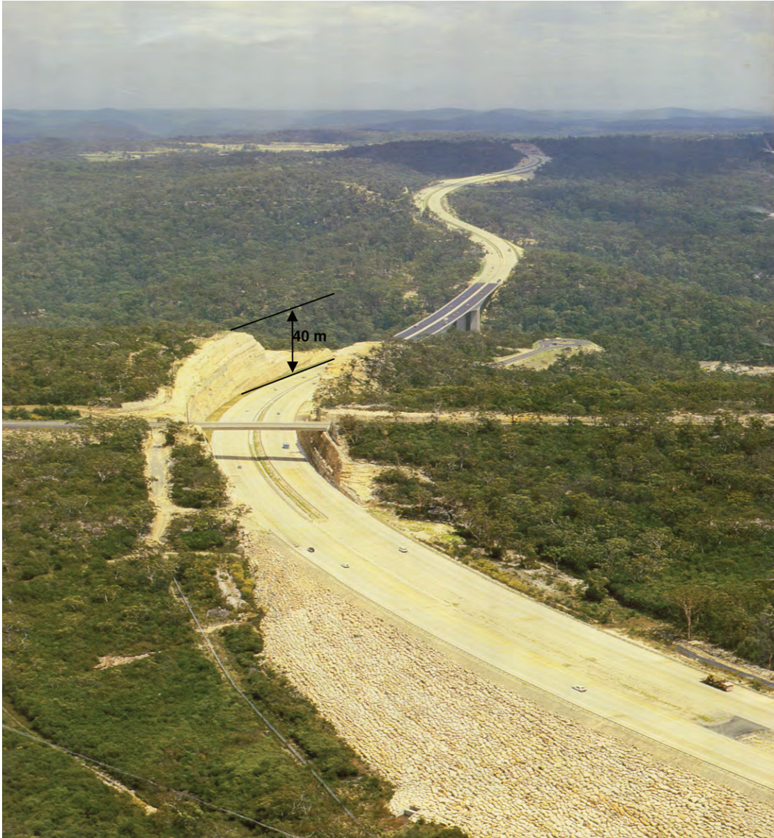
Figure 13 Photo of Sydney-Newcastle Freeway construction
